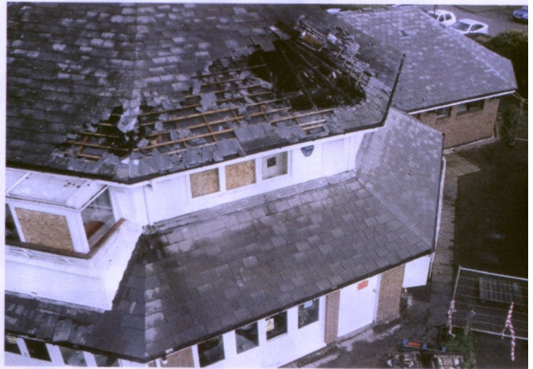
Grease in a kitchen extract system caused a fire at these premises
