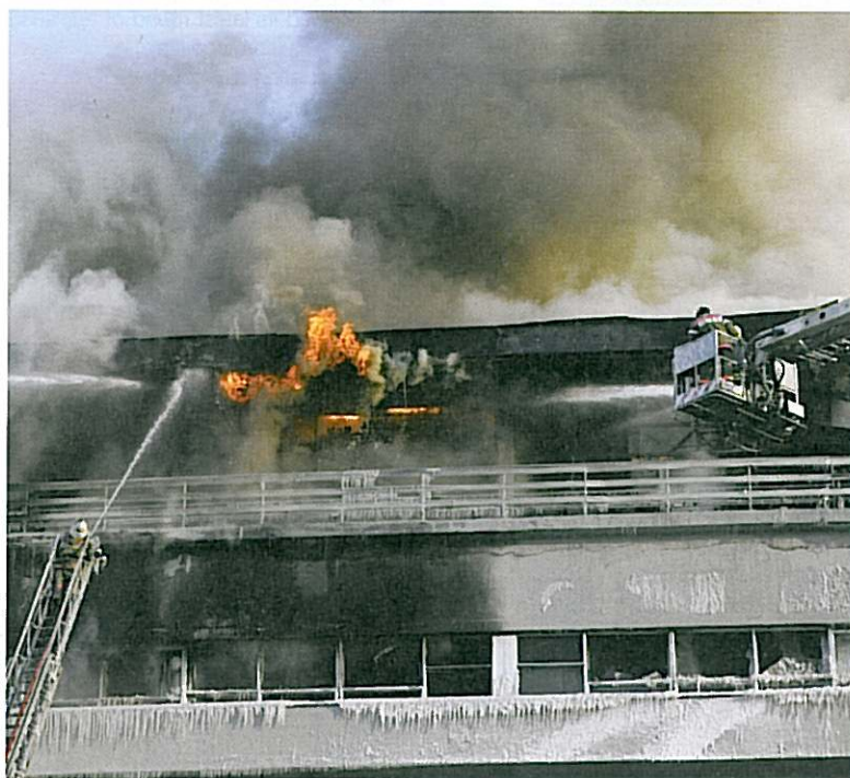
If fire regulators find no access doors in the ductwork, building owners could face prosecution
