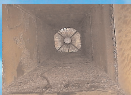
Kitchen grease extract ducts (pre-clean)
